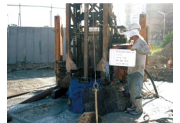
| Geo-thermal electricity system 3 |
